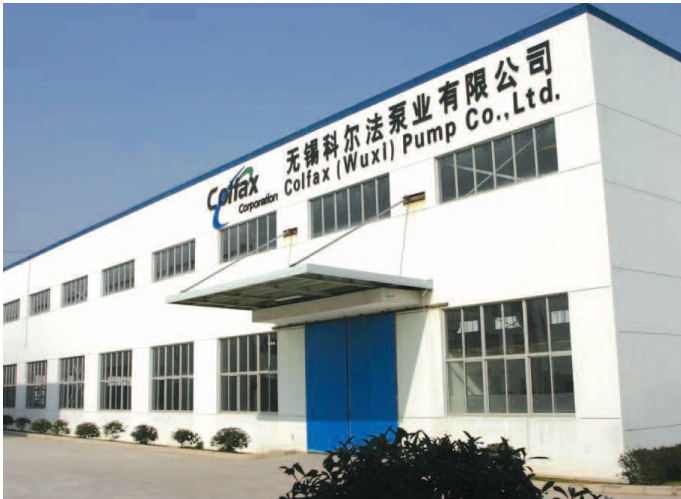
Colfax manufacturing and service centre in Wuxi, China
