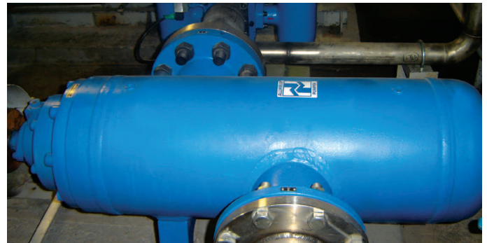
Allweiler SM three-screw pump installed on site
